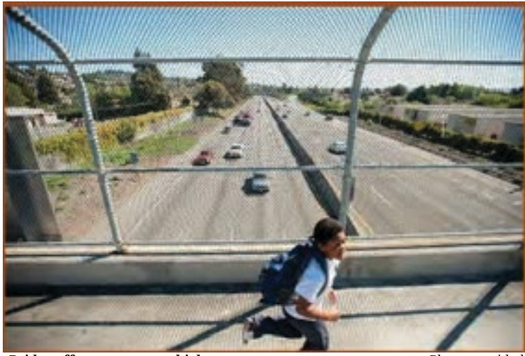
Bridge offers access over highway.
